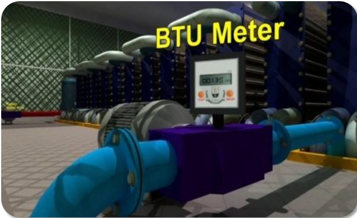
Figure 2: BTU Measurement Infrastructure.
