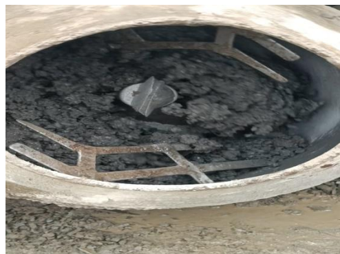
Fig. 6 Mixing of material in concrete Mixer
